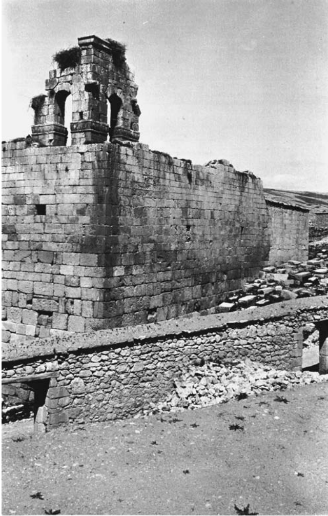
Fig. 2.6.7 Southern façade of the Church of Yoldath Aloho
